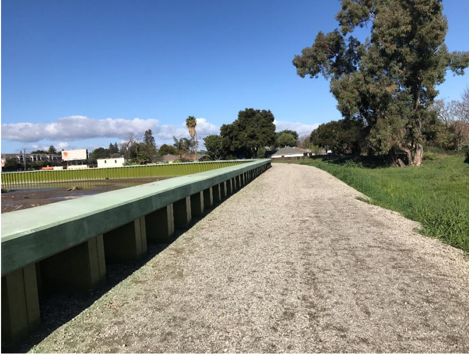
Figure 2-9. Example Sheet Pile Floodwall
