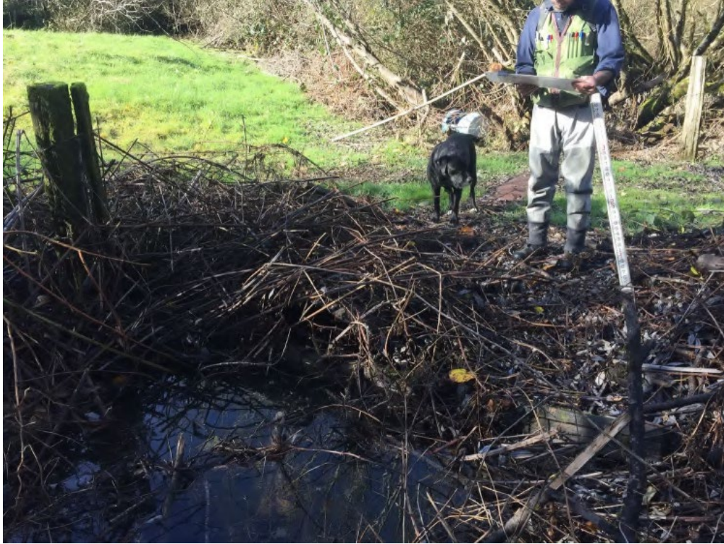
Figure 11. Crossing 2 (looking downstream at inlet) showing debris jams at inlet.
