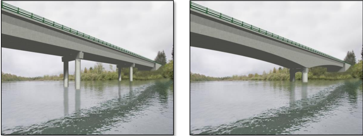
Figure 1-4. Uniform Soffit (No Arch Between Piers and Constant Bridge Depth) on Left and Parabolic Soffit (Arched Between Piers With Variable Bridge Depth) on Right
