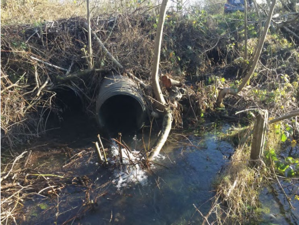
Figure 15. Crossing 4 (looking upstream at outlets) with two exposed outlet pipes. Other two outlets are not visible and are hidden behind blackberry vegetation.
