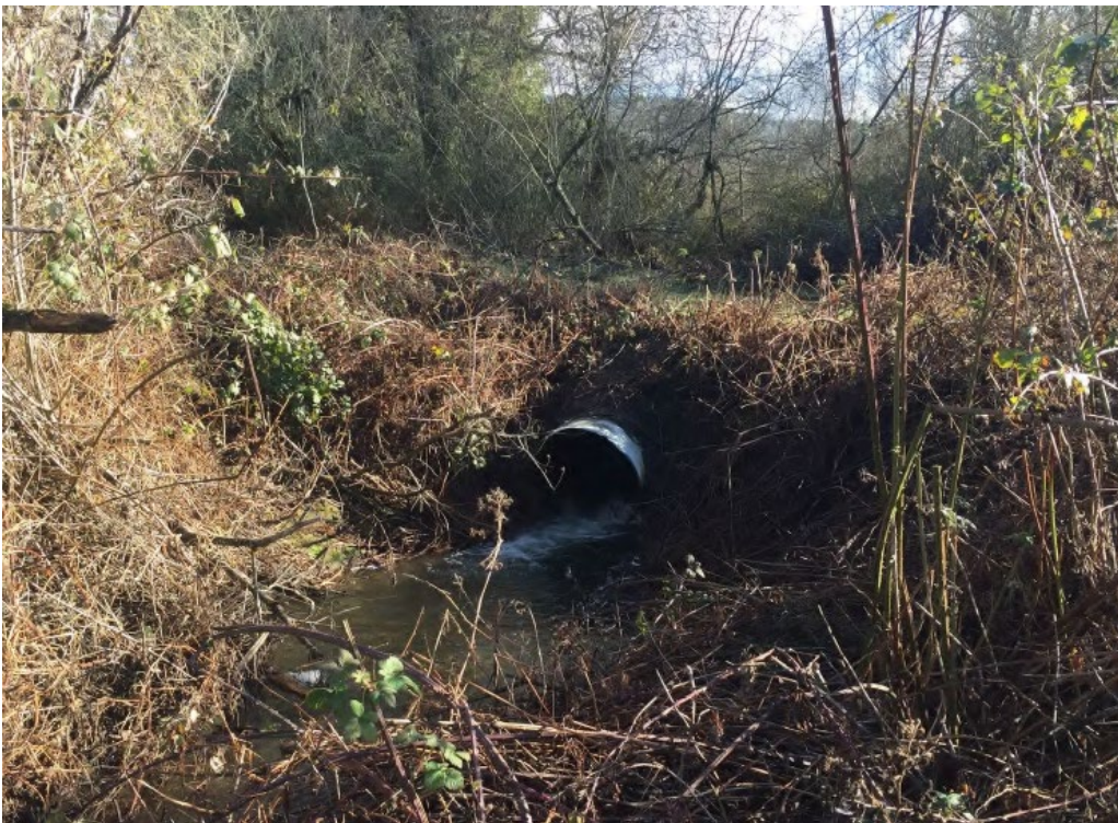
Figure 8. Crossing 1 (looking upstream at outlet) through access road showing scour pool.
