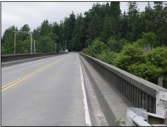
Photo 2. Looking north, non-standard concrete bridge rails, narrow shoulders (1-foot), and narrow elevated maintenance walkway (21-inches) are “functionally obsolete” elements.
