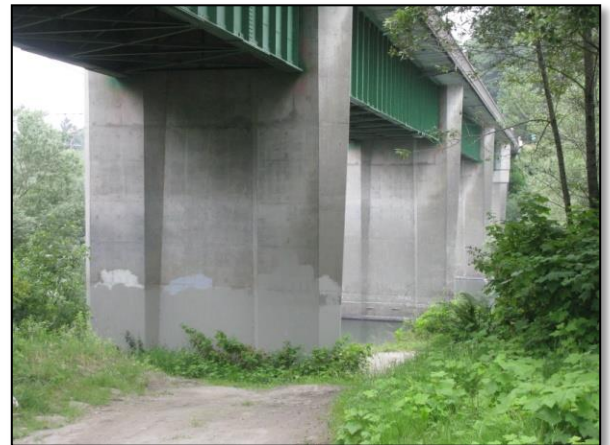
Photo 3. Existing painted green steel girders and concrete piers spanning the Smith River; looking north from the southern river bank.
