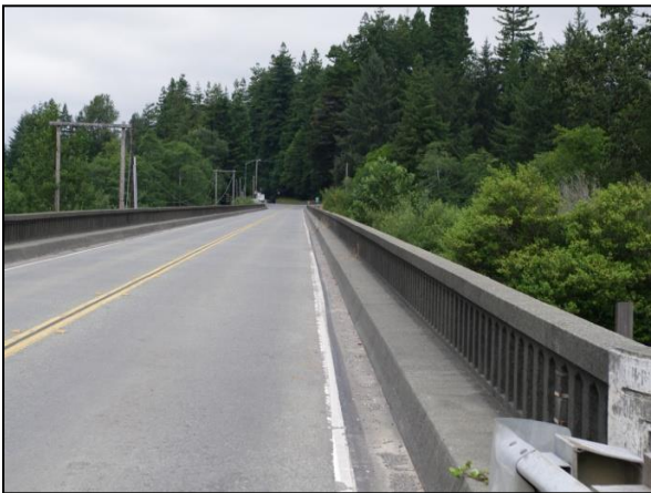
Photo 2. Looking north, non-standard concrete bridge rails, narrow shoulders (1-foot), and narrow elevated maintenance walkway (21-inches) are “functionally obsolete” elements.
