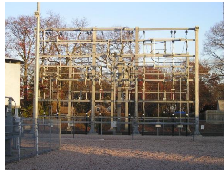
Figure 17 Traction Power Substation Overhead Contact
