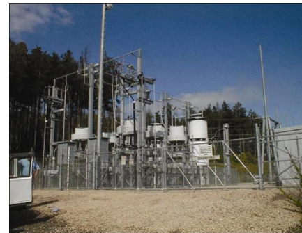
Figure 16 Traction Power Substation
