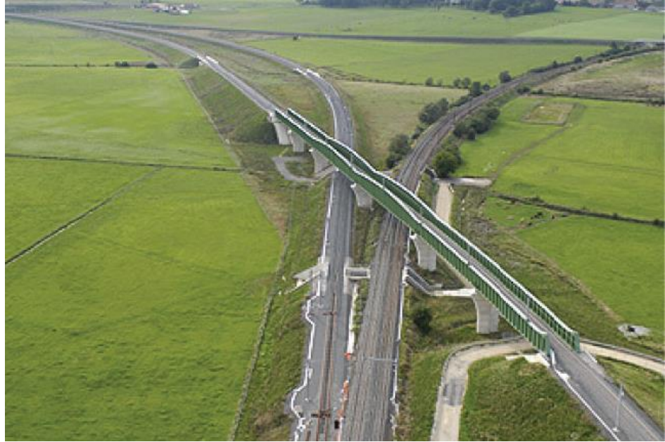
Figure 15 Photograph Showing an HSR Wye Configuration with One Wye Leg Crossing Another
