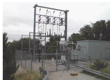
Figure 19 Paralleling Station
