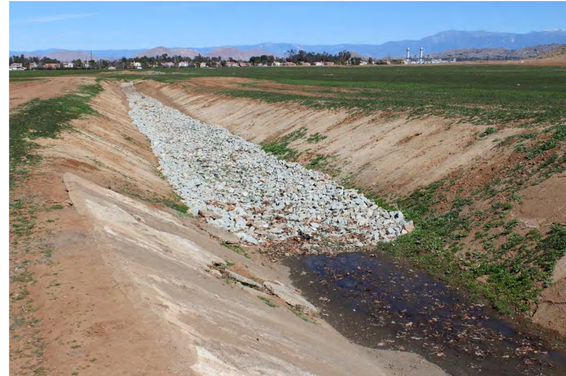
Photograph 2: View of the drainage ditch looking north where the ditch transitions from a concrete-lined ditch to an earthen ditch with un-grouted rock.
