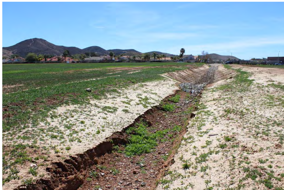
Photograph 3: View of the drainage ditch looking south, depicting where the ditch transitions from a deeper earthen channel (with rock lining) to a shallower earthen channel.
