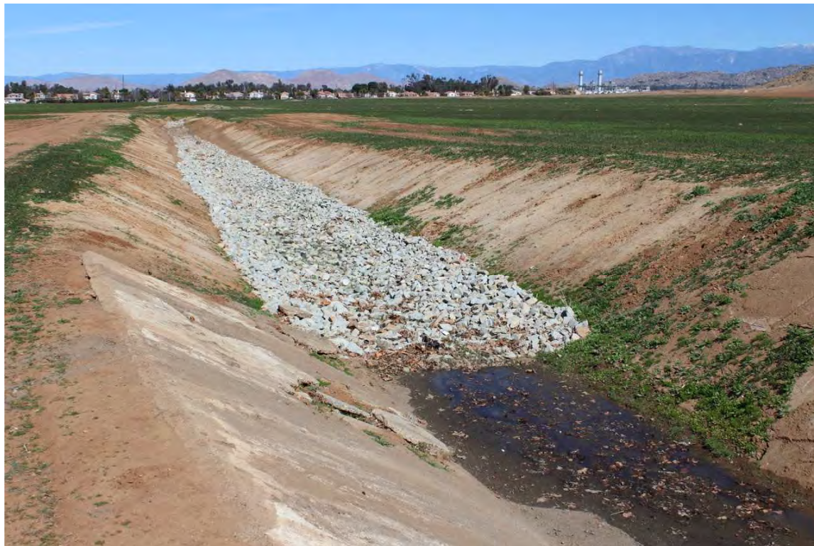
Photograph 7: View of the drainage ditch looking north where the ditch transitions from a concrete-lined ditch to an earthen ditch.
