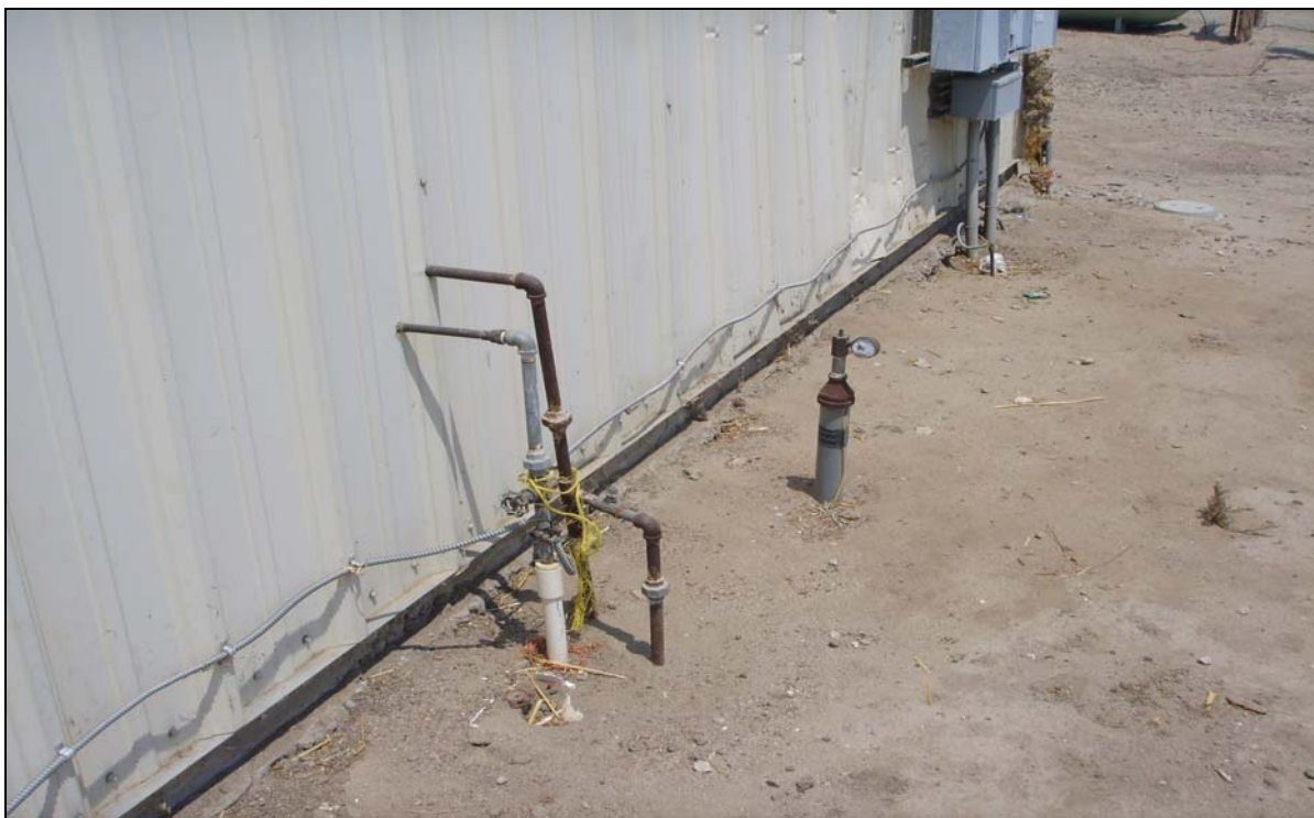
Photo 13. On the east side of the steel shop building are natural gas lines (left of center), an air compressor line (right of center), and electric circuit boxes at top right.
