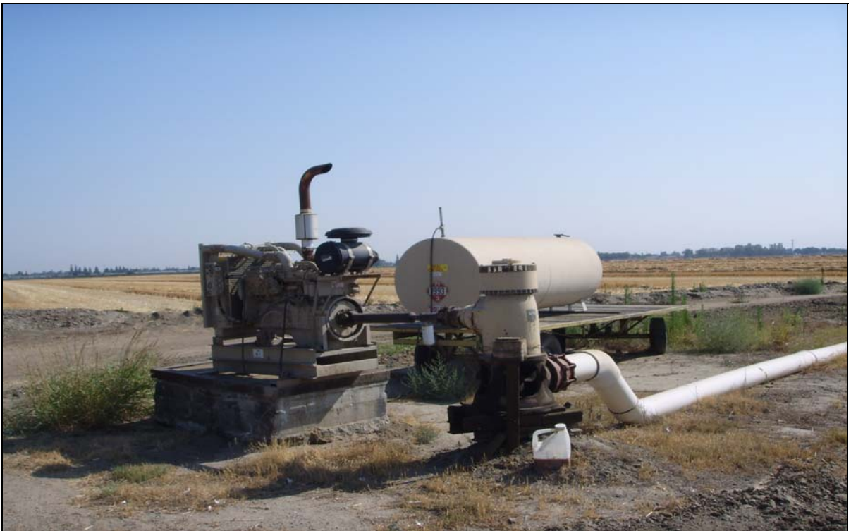
Photo 6. Northeast-facing view of the northwest irrigation well with diesel engine and trailer-mounted AST, located in the northwest corner of the project site.
