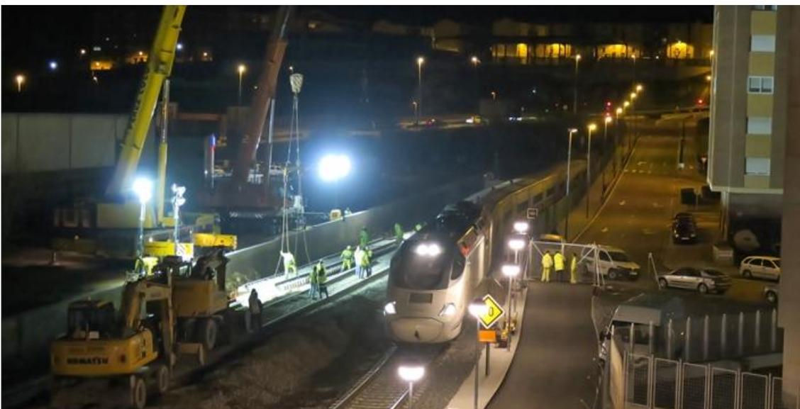
Figure 11. Assemble of a pre-assembled turnout with cranes
