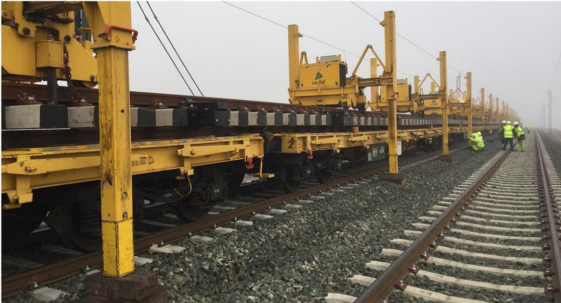
Figure 10. Transportation of a pre-assembled turnout
