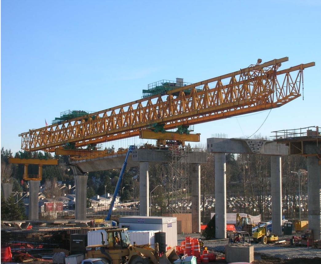
**Figure 4-6 Precast Segmental Construction**
