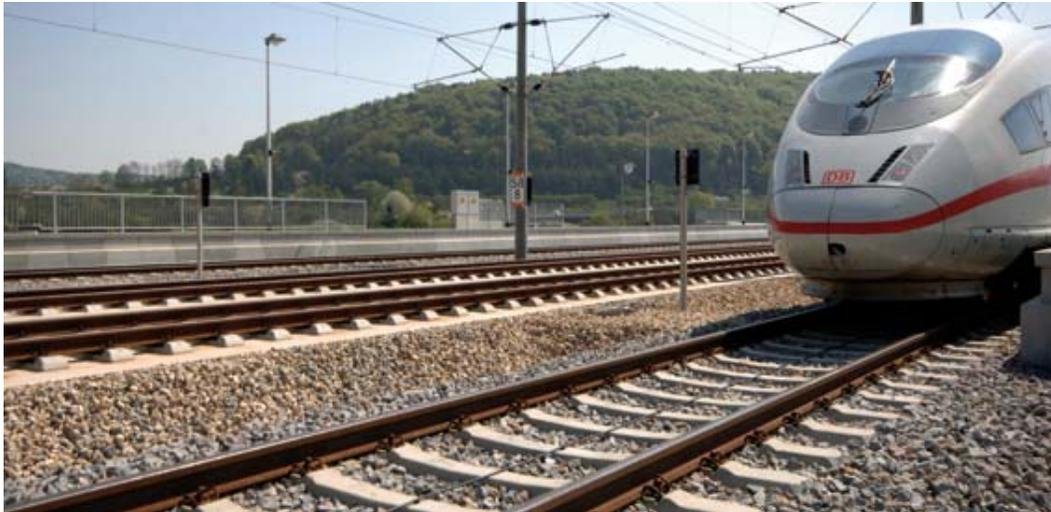
**Figure 4-13 Ballast Track - Schotteroberbau**
