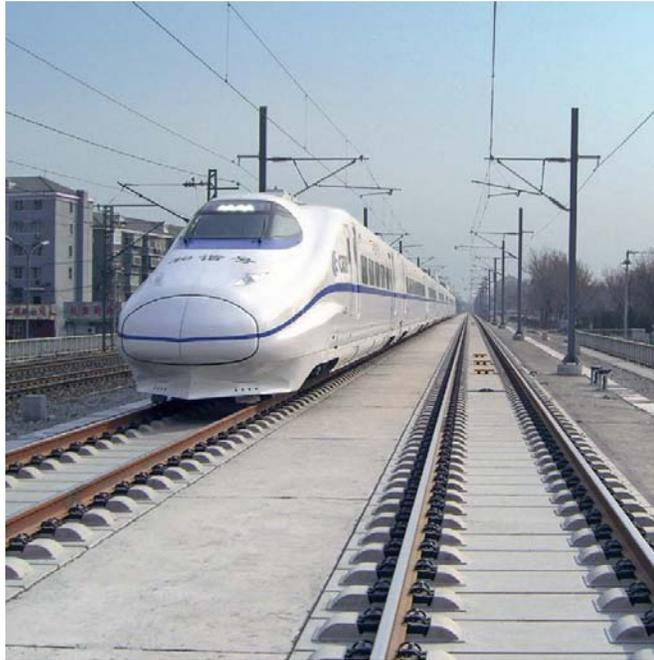
**Figure 4-16 Slab Track - China HSR**
