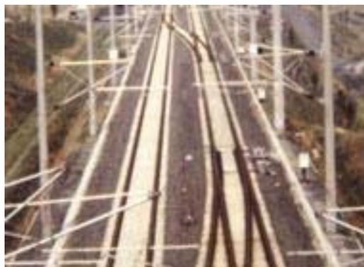
**Figure 4-15 Ballast Track Turnouts**
