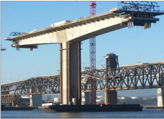
**Figure 2-72 Balanced Cantilever Segmental Construction**
