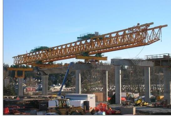
**Figure 2-71 Span-by-Span Precast Segmental Construction**
