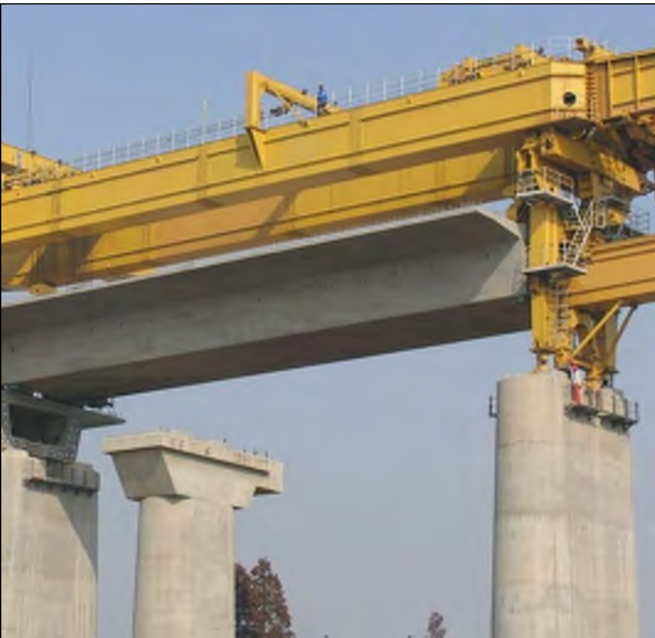
Appendix A Monterey Highway Viaduct Typical Section Installation – Full Span Precast
