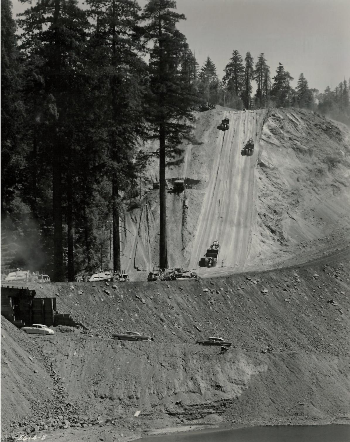
**Figure 7. Representative photo of historic US 101 construction near Dyerville. Note the re-routed portion of the South Fork Eel River in the foreground. (State of California, Division of Highways, 1956)**
