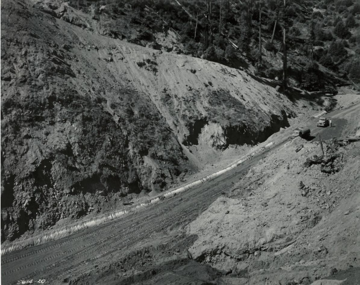
**Figure 8. Representative photo of historic US 101 construction near Dyerville showing culvert installation. For scale, two trucks and a worker can be seen at the center of the right side of photo. (State of California, Division of Highways, 1956)**
