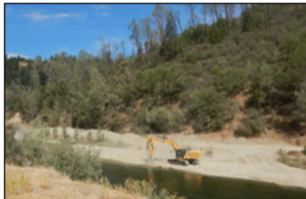
Photo 1. Gravel augmentation near Trinity River Hatchery in summer 2021. 6
