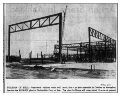
Plate 3. Photograph of Trailmobile manufacturing plant under construction, showing triangular framing pattern used throughout the building structure (Source: Oakland Tribune 1960).
