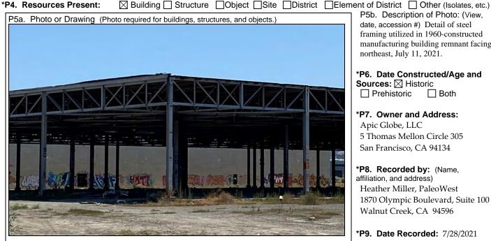
P5b. Description of Photo: (View, date, accession #) Detail of steel framing utilized in 1960-constructed manufacturing building remnant facing northeast, July 11, 2021.
