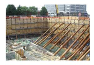
Rakers and tiebacks provide temporary support during construction.
