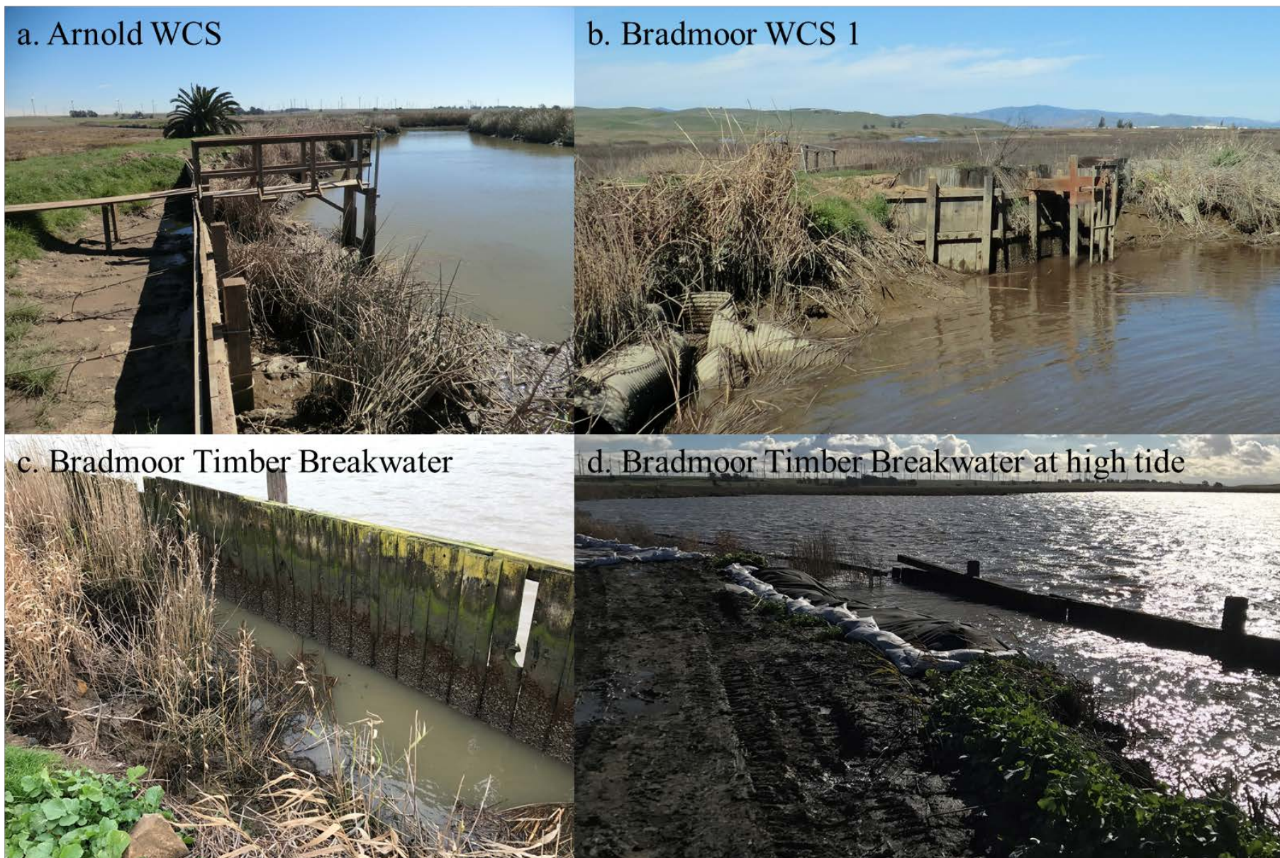
Figure 2-7. Typical Water Control Structures and Timber Breakwater
