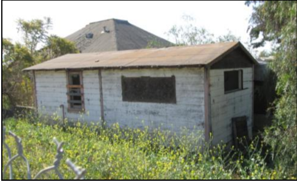
Figure 18: Guest house/bunkhouse situated to the immediate northeast of the main house. View looking southeast. One of the original Victorian-era windows is on the left hand side of the north elevation, while one of the new, unfinished openings is visible in the upper façade of the west elevation.
