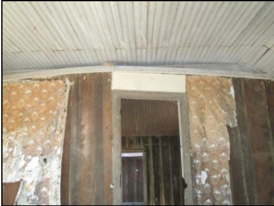
Figure 14: Interior walls and ceilings of the small residence. Note that both the walls and ceiling are clad with either flat boards (walls) or narrow tongue-in-groove panels covering the ceiling. Also note that the ceiling is canted downwards where it meets the side walls of the room, and the top of the interior wall (with the scraps of remaining wall paper) is framed as an arch instead of meeting the ceiling. View looking from south room to the north.
