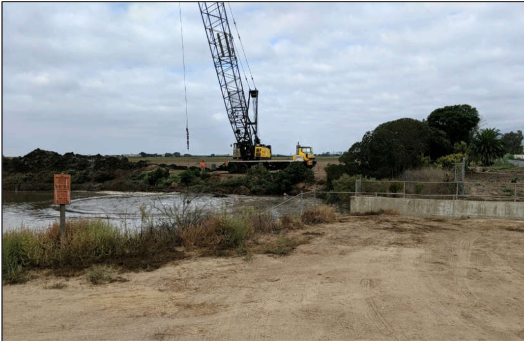
Figure 3-5. Drag-line Desilting Operation on Santa Monica Creek
