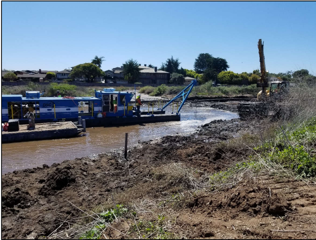
Figure 4-3. Hydraulic Dredging Operation at the Marsh
