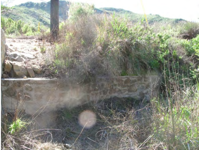
IMG_0167. Partially buried rock and concrete retaining wall, facing southwest.
