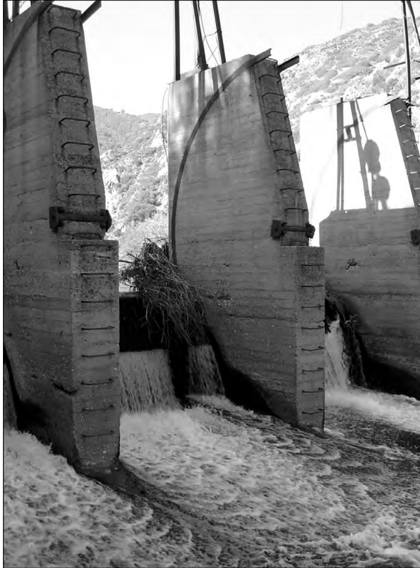
Figure 8. View from the edge of the spillway apron, showing the pivot point locations for the radial-arm gate supports and the curved, metal bearing plates for the gates.
