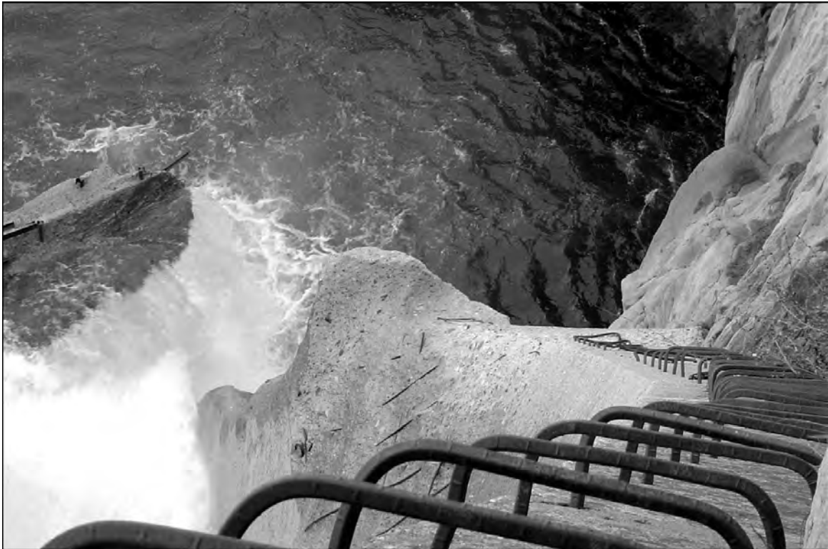
Figure 13. View down the south side of the spillway wall shows erosion of concrete in this portion of the spillway. Steel rungs that lead down this wall are in relatively good condition.
