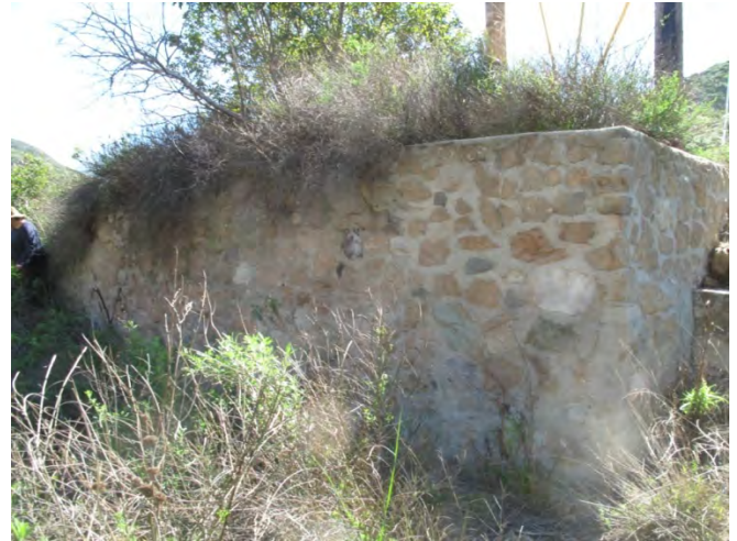
IMG_0168. Rock and concrete power pole retaining wall, facing southeast.
