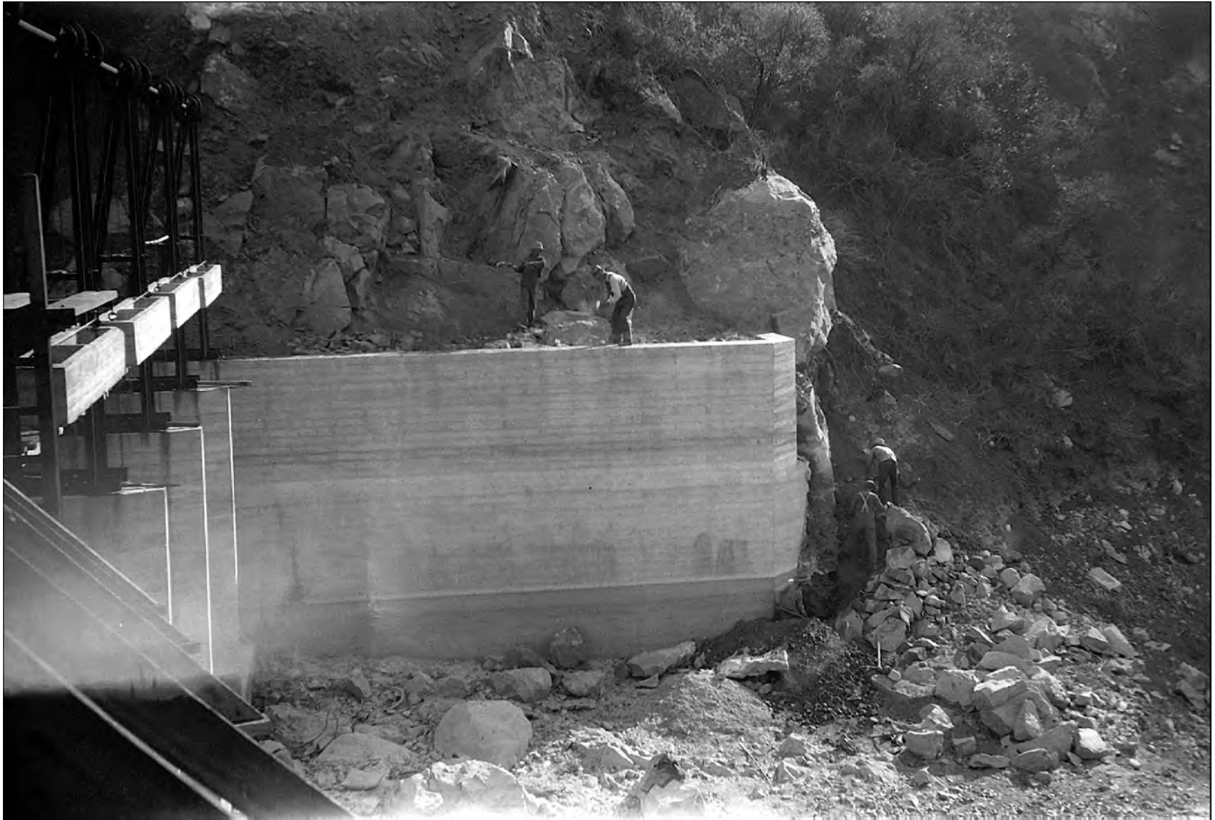
Figure 2. Construction of the upstream (reservoir) side of spillway, ca. 1926. Note the steel rails used to form the metal framework for raising and lowering the radial gates (photograph courtesy of the Malibu Lagoon Museum/Historic Adamson House, No. MD-2).
