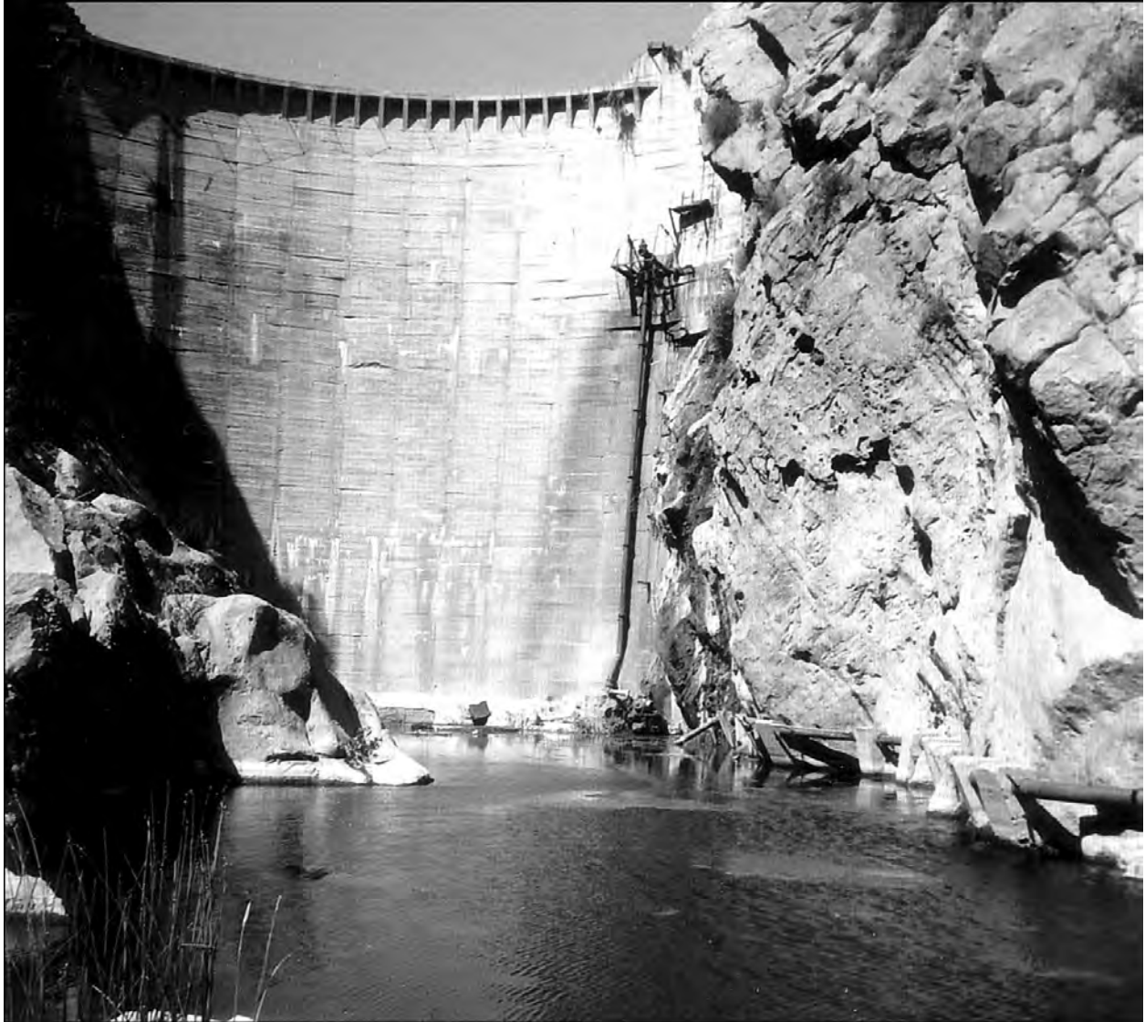
Figure 5. Dam wall, viewed north from Malibu Creek, 1966. The 8-inch distribution line can be seen exiting the dam roughly one-third down from the top. At the base of the dam, this connects to the horizontal distribution pipe attached to the canyon wall (Mario Quiros photograph, courtesy of Louis T. Busch).
