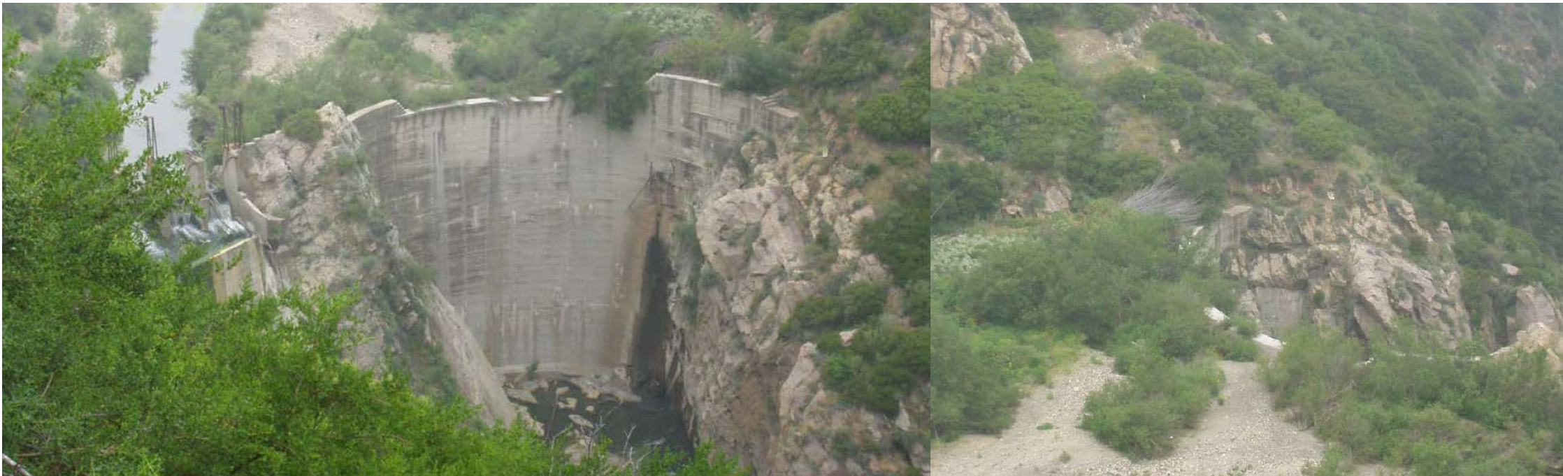
Clockwise from left: View of the downstream face of the dam, left and right abutments, and spillway. View of the upstream face and crest of the dam. Sediment has deposited on the upstream face almost to the top. View of the upstream side of the spillway.
