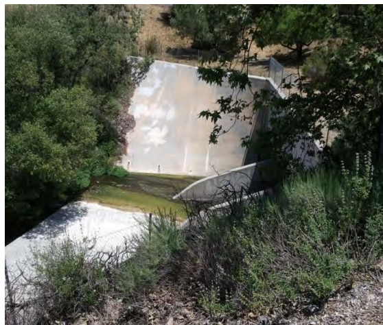
View upstream from Lost Hills Rd. showing wing walls.
