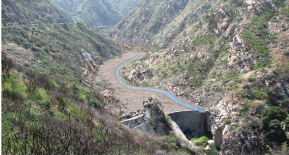
Figure 5.7-2 - Rindge Dam Mid-Point of Construction - 50% Removal
