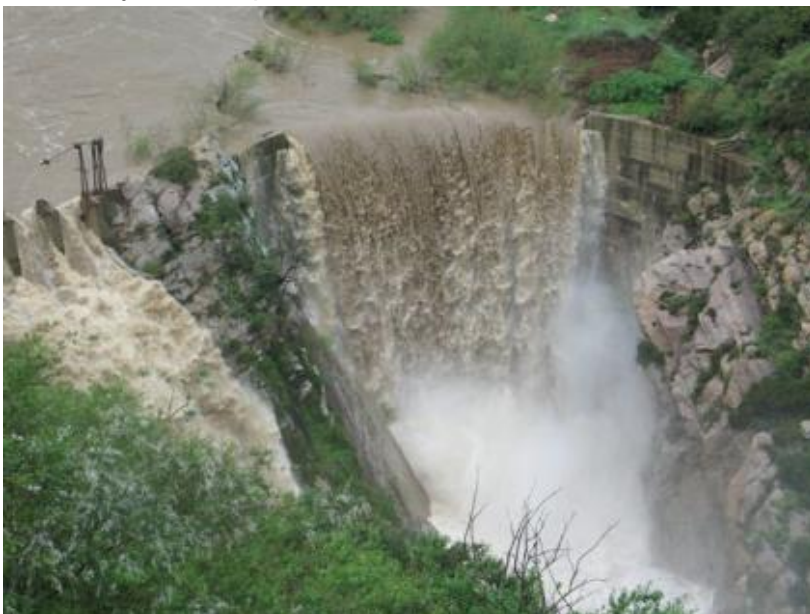
Photo 1.10-4 – Rindge Dam Arch & Spillway – 2005 Storm (5-10 yr event)
